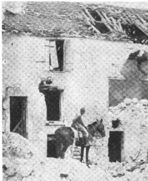
Wrecked building at Chateau-Thierry. The horseman in the foreground is Lt. H. J. Sanders of Racine. The picture was taken July 30, 1919.
